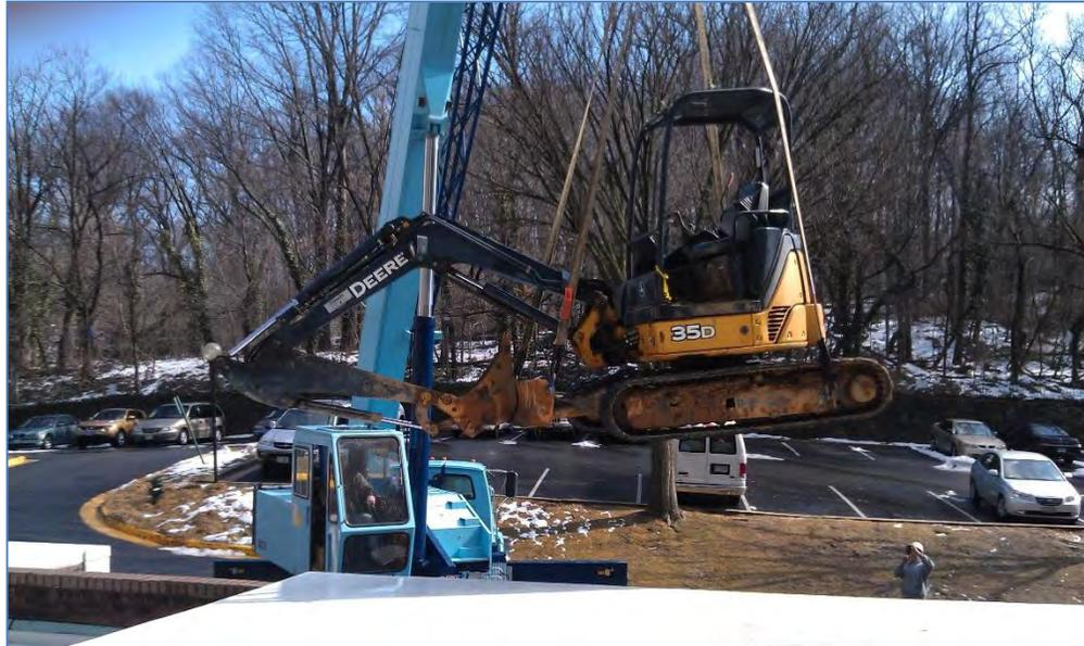
The leak was found and repaired on Thursday February 20<sup>th</sup>. It was approximately eight (8) feet below the surface and was on a 6” fire service line. The size of the leak was estimated to be 30 gallons a minute. Nice work **Rick**!
